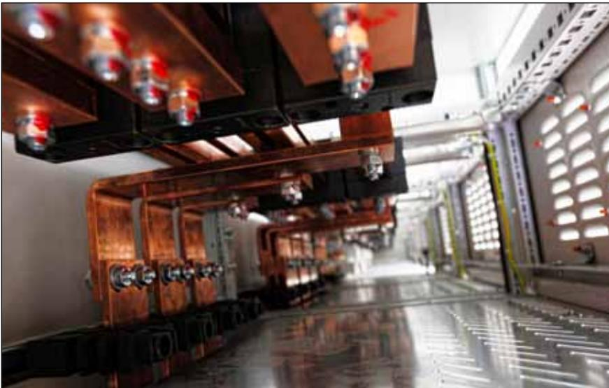
Instead of complex wiring in the floor, a Rittal Maxi-PLS busbar system laid in the container roof distributes power to the individual switchgear panels.
