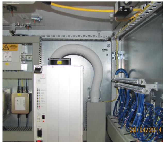
▲ Fig 2. The new module comprises the so-called FMT24S machine processor (left) and the bridging EPRO Interface Board (EIB) developed specially for the purpose. The connections for the EPRO valve drivers and the control panel are located on the front plate and all others on the rear. The rack can be tilted forward for installation.
