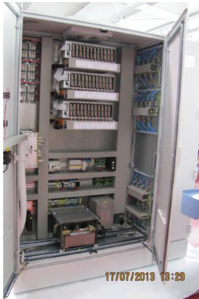
▲ Fig 3. Neat and tidy: this [new] control cabinet still houses an original EPRO control (left). Each retrofit should also include new cables, depending on the system's age and condition. They could become brittle over the years and lead to faults in view of the harsh production conditions prevailing in glassworks.
