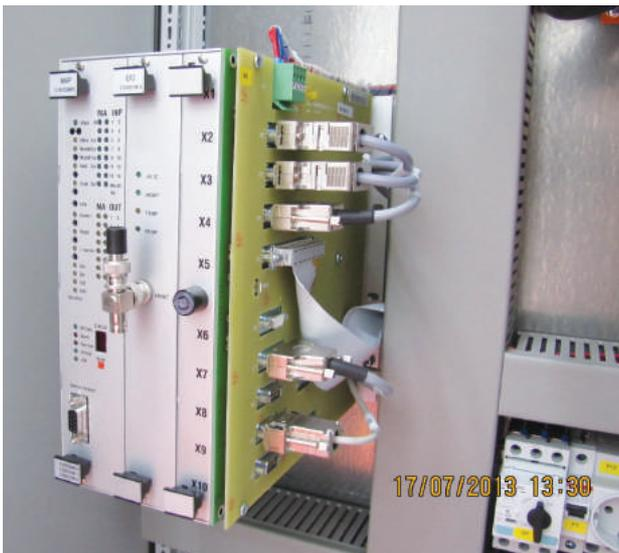
▲ Fig 1. The central processor rack containing the ArcNet module is removed from the control cabinet along with the old connections for the control panel and the flat cables for the valve drivers.
